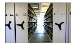
Spacesaver mechanical assist high-density mobile shelving. The library repurposed some of the original glass floor tiles and used them as a wall on the ground level. The use of high-density mobile shelving enabled the library to consolidate the collection from their seven-tiered central system onto just three interior mezzanine-like floors, plus the basement level of the library. Not only does the new stack space meet fire and seismic codes, it is brighter and easier to navigate.
